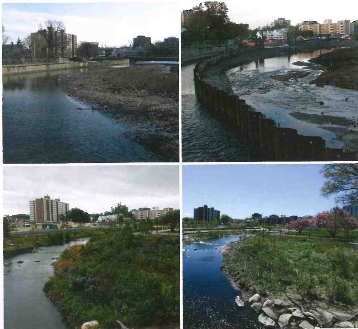
LEFT Fifteen-foot flood walls were built in 1922, but the channelized river continued to overflow due to urbanization. Re-establishing the river's natural habit has mitigated much of the flood risk.
