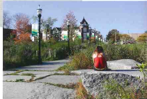
BELOW Boulders excavated from the site were used for seating and paving.
