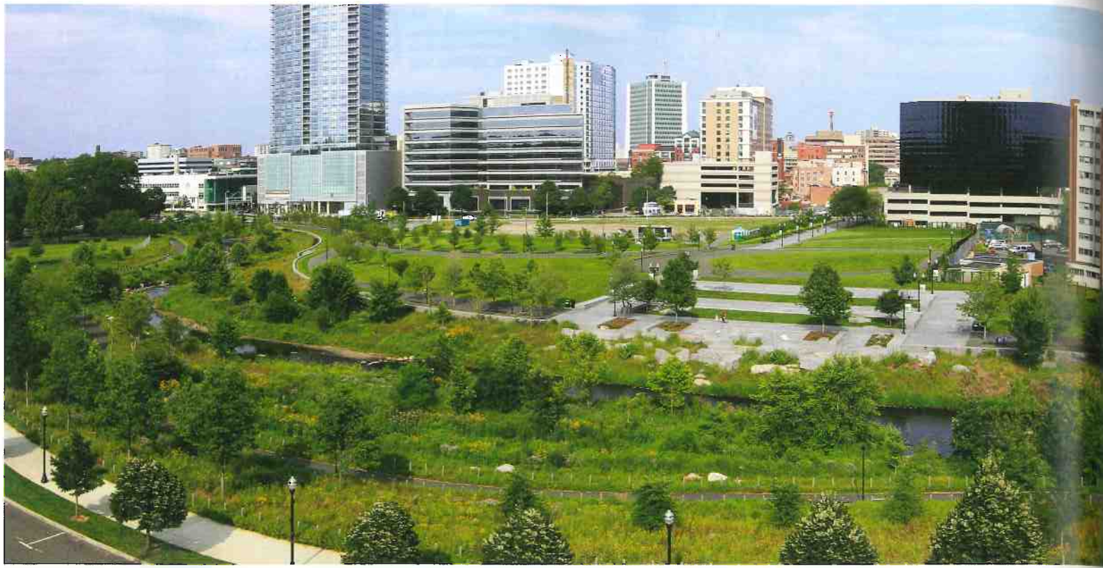
BELOW Riffles and pools replaced the dam and concrete channel.
